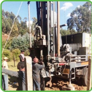
Setting a drilling rig on site
