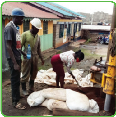
Installation of gravel pack into the borehole annular space.
